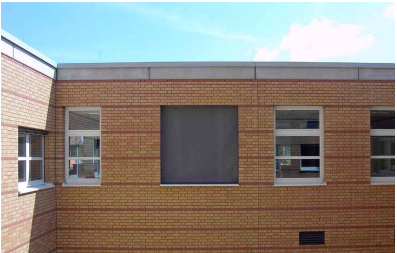
Sealing a facade at Hospital Greifswald
