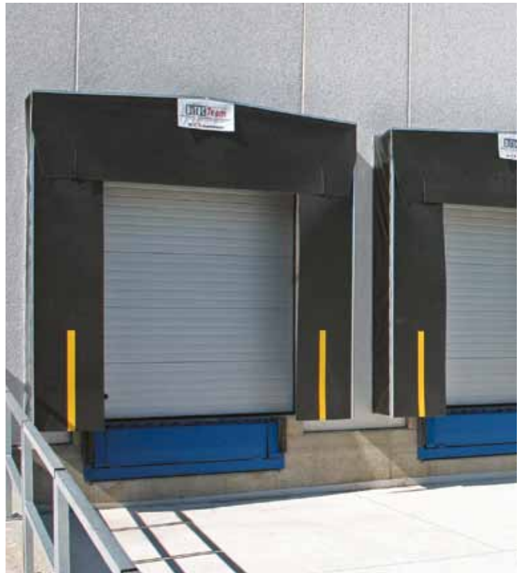
Bay Loading bays for logistic operations.
